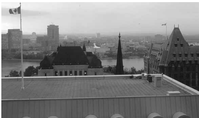
Figure 5. Light colored paving on low-slope roofs reflects light saving on air-conditioning costs while protecting the waterproofing.
