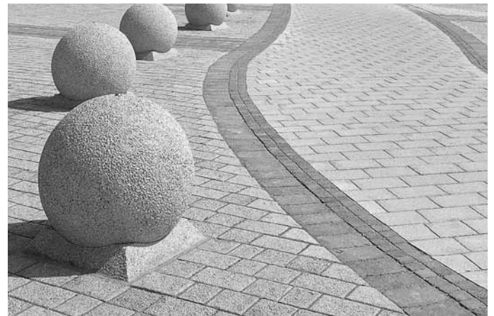
Figure 4. Light colored paving units reflect light and help reduce micro-climatic temperatures.
