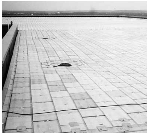
Figure 4. Some ballast-type slabs for roof decks are made with lightweight concrete materials. They can be joined with tongue-and-grooves and/or with connectors to resist wind uplift. This is one of several designs available.
