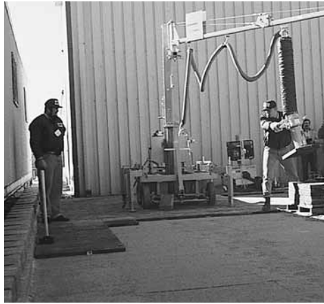
Figure 20. Vacuum assisted mechanical equipment for installing paving slabs.
