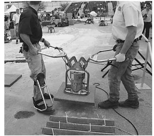
Figure 20. Vacuum assisted mechanical equipment for installing paving slabs.
