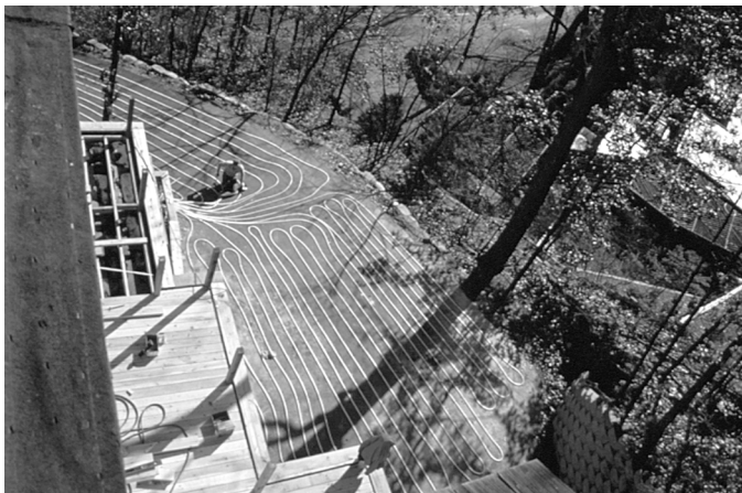
Figure 6. Experienced electrical and plumbing contractors should install snow melting systems.
