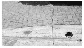
Figure 3. Ramp pavers changing angle.
