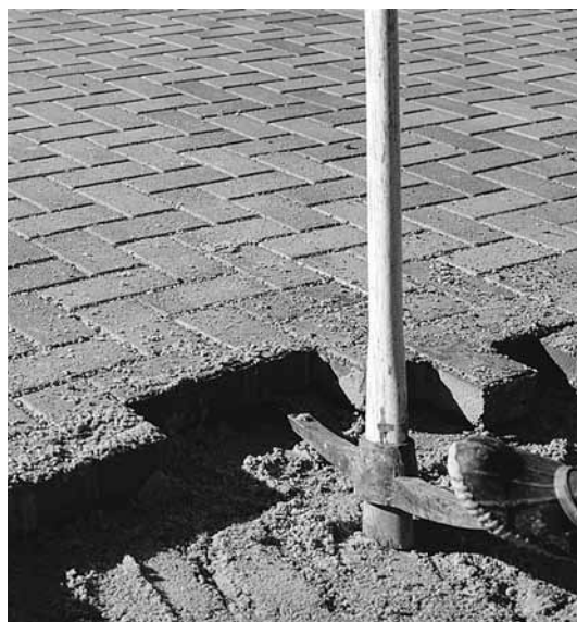
Figure 6. Prying out the remaining pavers
