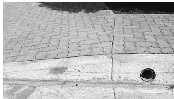
Figure 3. Ramp pavers changing angle.
