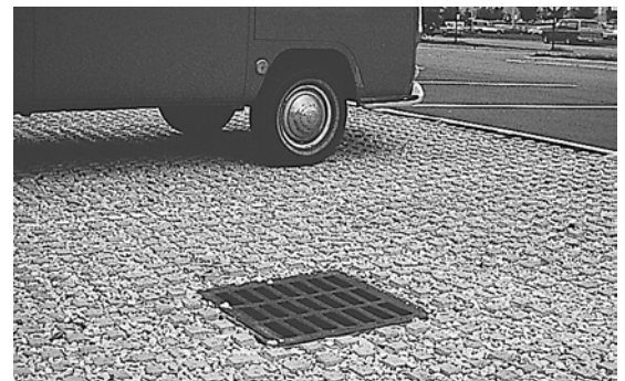
Figure 18. Concrete grids with aggregate in the openings
