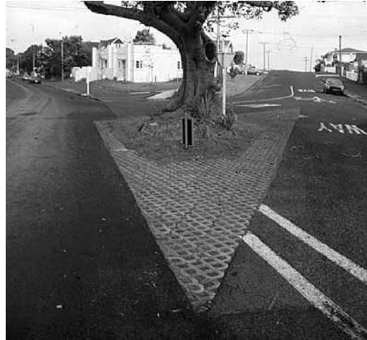
Figure 13. Air for tree roots and a warning for drivers
