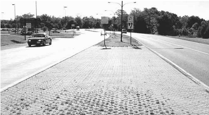
Figure 6. Roadway median crossover
