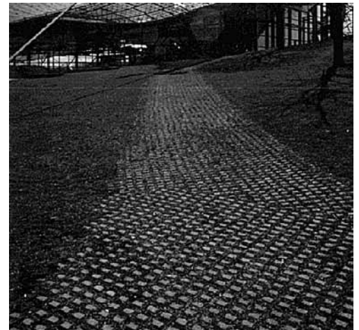
Figure 7. Service access lane
