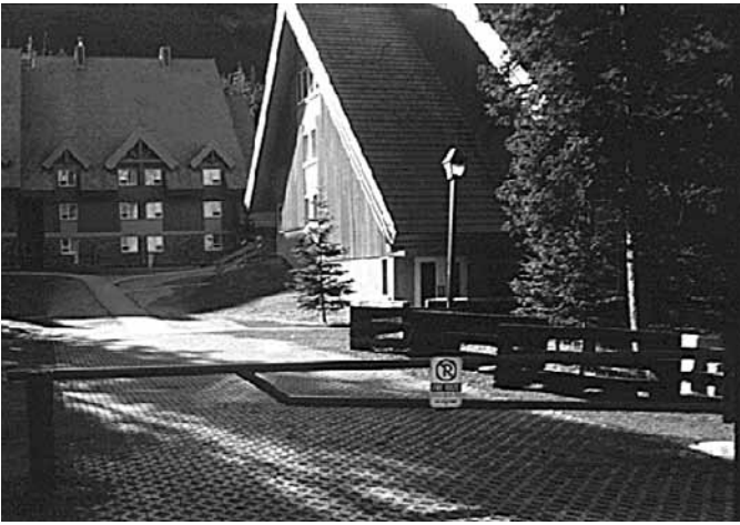
Figure 8. Emergency access lane for fire trucks
