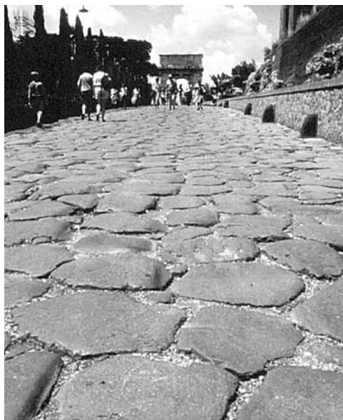
Figure 1. The Roman Appian Way: early interlocking pavement
